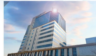
SOUTH KOREA. HEADQUARTER. MCNEX TOWER
